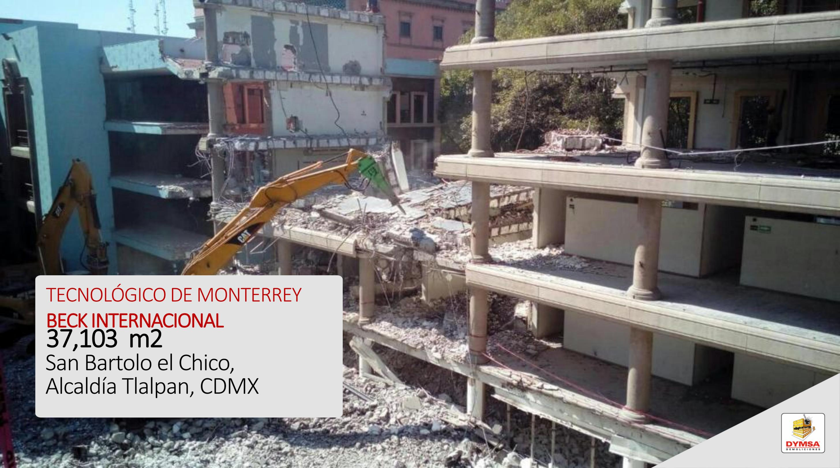
A photograph showing the demolition of a multi-story building. A yellow excavator with a green hydraulic breaker attachment is positioned in the center, actively demolishing a concrete structure. To the right, a partially demolished building with a grid of concrete columns and beams remains standing. The ground is covered in rubble and debris. In the background, other buildings and utility poles are visible under a clear blue sky.
